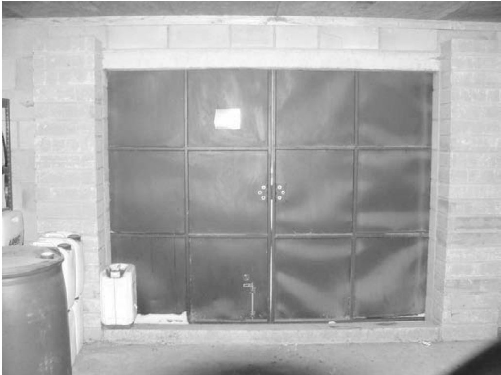
Figure 6: Interior of store showing wide, lockable steel doors for delivery/ removal of products and wastes on pallets.
