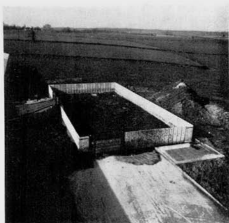
Fig. 1: Safe storage conditions
